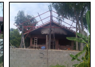
THE RETAINING WALL IS UP, BACK-FILL DIRT EXPANDS SPACE & THE STRUCTURE GOES UP
