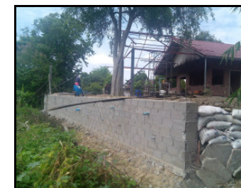
THE RETAINING WALL IS UP, BACK-FILL DIRT EXPANDS SPACE & THE STRUCTURE GOES UP
