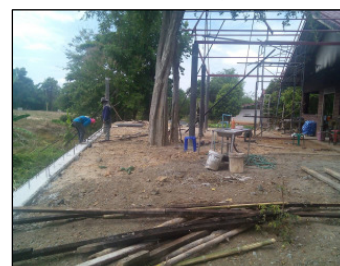
THE RETAINING WALL IS UP, BACK-FILL DIRT EXPANDS SPACE & THE STRUCTURE GOES UP
