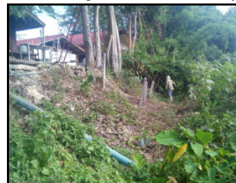
CLEARING THE DROP-OFF DRAINAGE AREA
