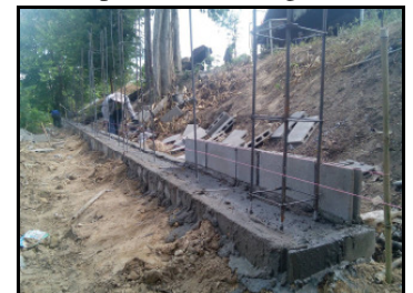
A SOLID CEMENT FOUNDATION FOR THE WALL
